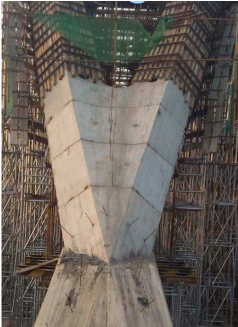
Figure 10. Fasteners dismantling after pouring
