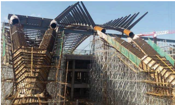
Figure 8. Installation on site
